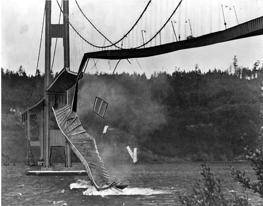
Figura 1.2 – Ponte de Tacoma Narrows.
